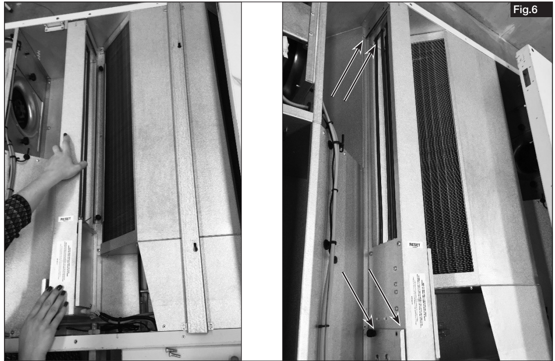
6. Connect electrical auxiliary heater via plugs (see Fig. 7).
