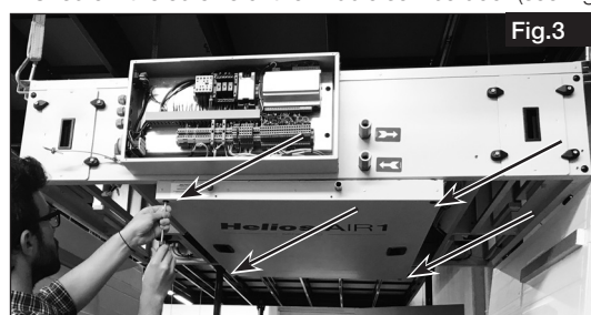
3. Remove service door in direction of the terminal box (see Fig. 4).
