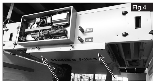
4. Remove support plate if necessary (see Fig. 5).
