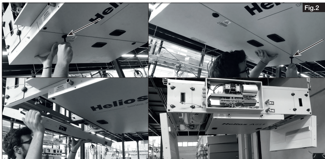
2. Unscrew the screws of the middle service door (see Fig. 3).
