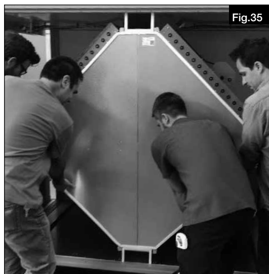
6. Carefully remove the cross-counterflow heat exchanger from the unit and set down safely (see Fig.35/Fig.36).
